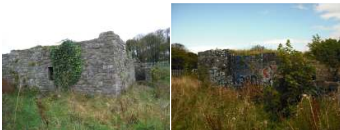
Rush Tower House November 2007 and August 2010
