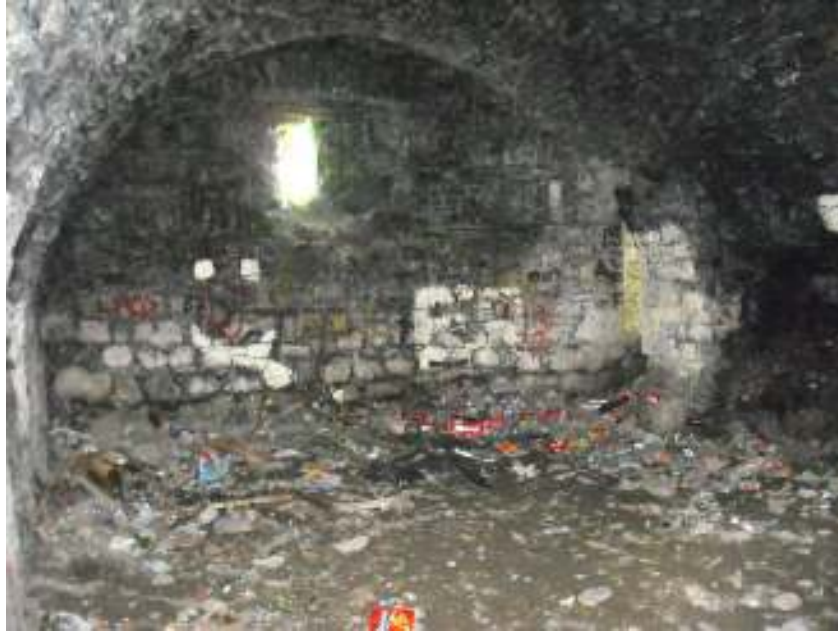
Internal view Rush tower-house
